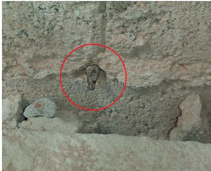
Corroded Joint Reinforcement
