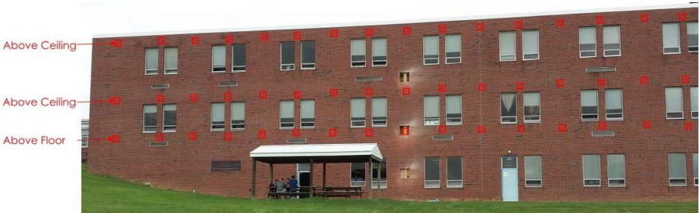
Figure 12: Typical Anchor Layout (Note: Other walls similar)
