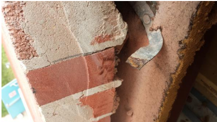
Failed Corrugated Wall Tie
